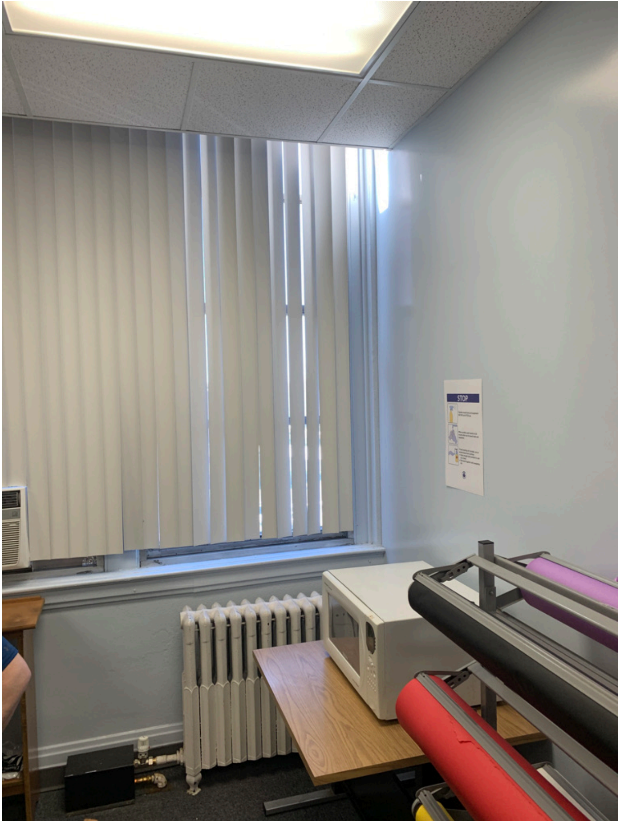
Radiators provide heat and the windows provide natural ventilation
